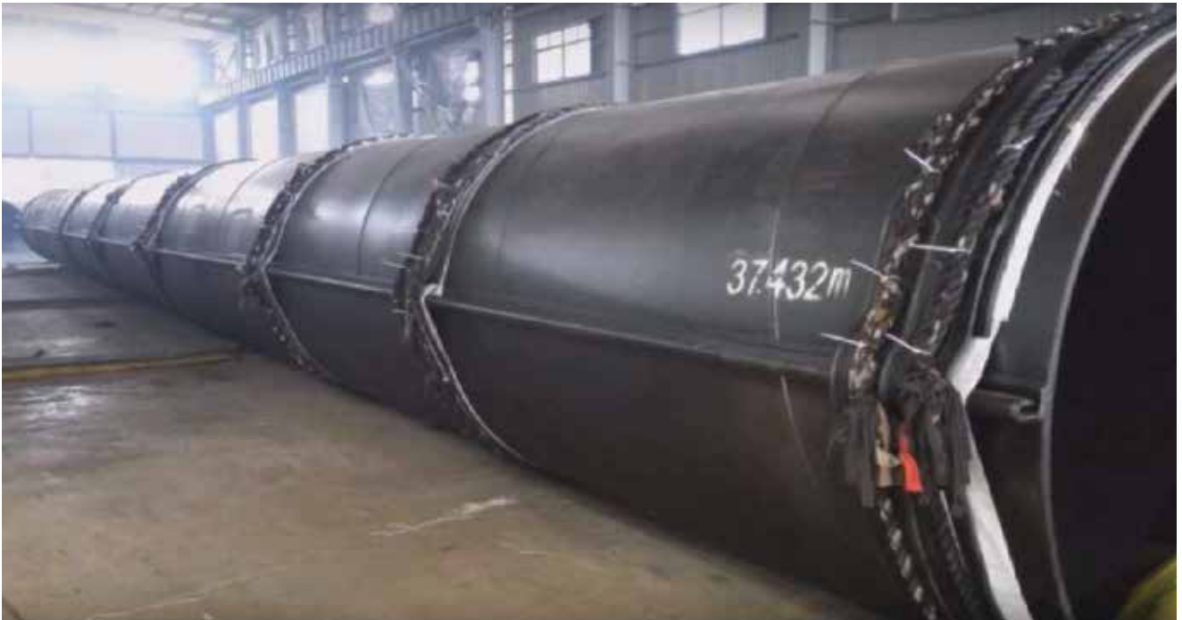
Painted, rope separator protected, with corner piles welded
